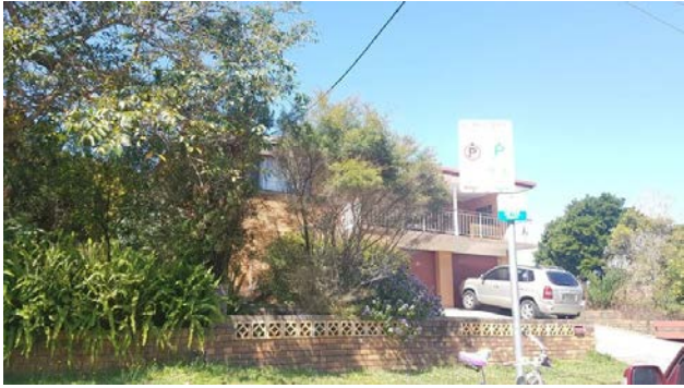
Existing dwellings No.137 and No.139 Jonson St
